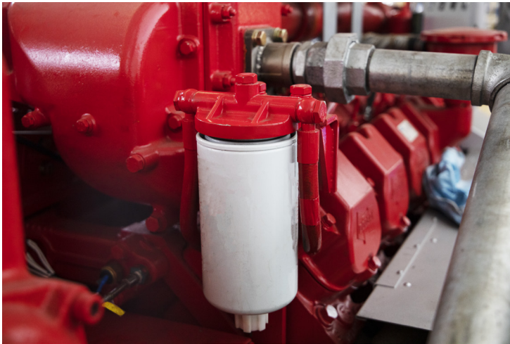
FIGURE 20 - FUEL FILTER
