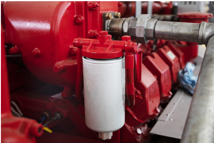
FIGURE 20 - FUEL FILTER
