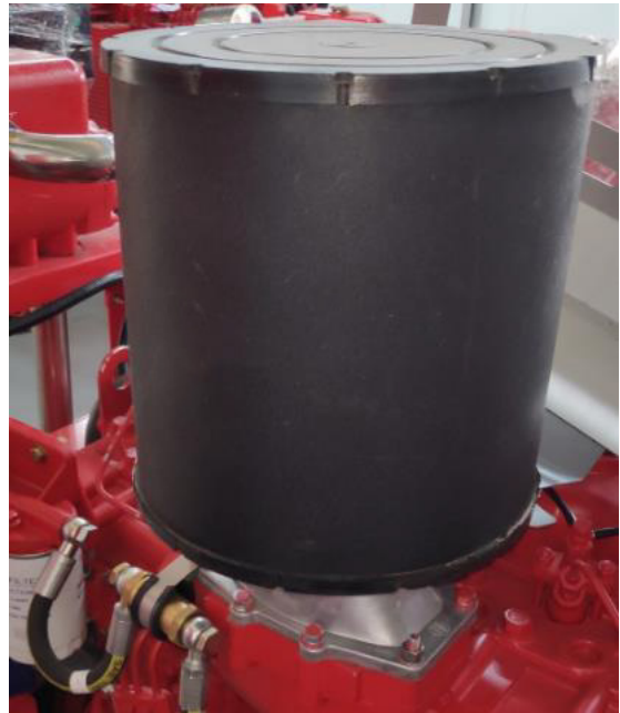
FIGURE 19 - AIR FILTER HOUSING
